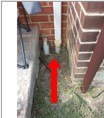
Gutter run-off into ground drain
